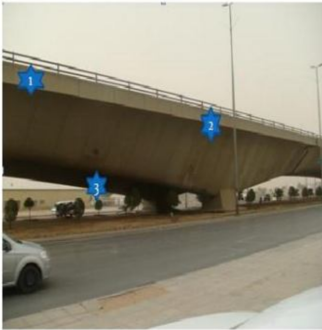
Fig 1.4 Placement of 3 sensors for real time
